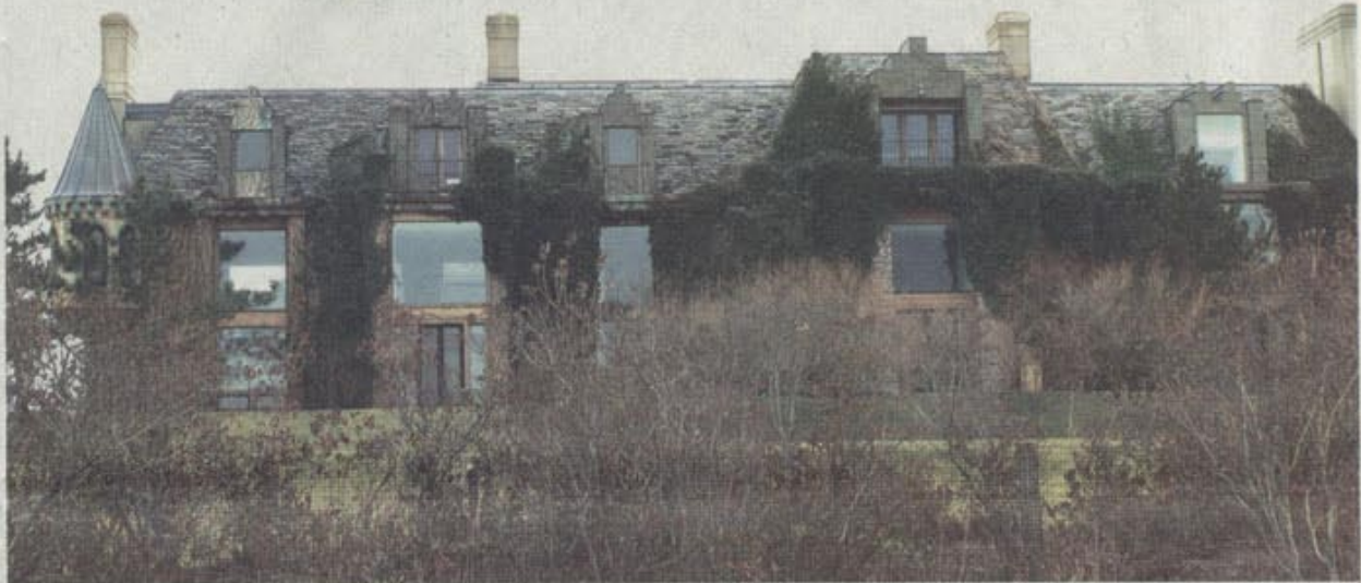
The controversial Dragon's Head, now owned by Calvin Klein, could be torn down and replaced with a smaller home.
