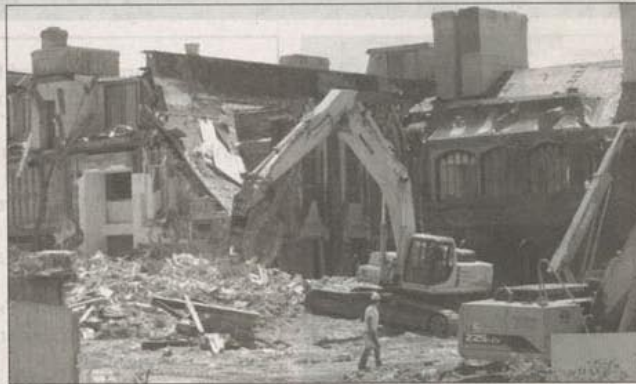
Demolition crews do their work on Dragon's Head last week.
